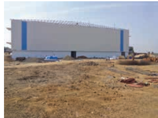
USED IN WAREHOUSE
